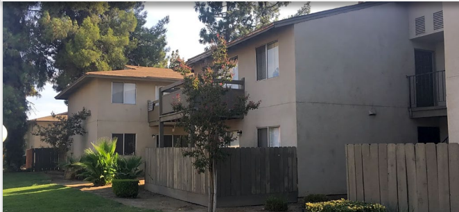
2120 Villa Ave, Clovis Ca, 93612 EDGEWOOD APARTMENTS
