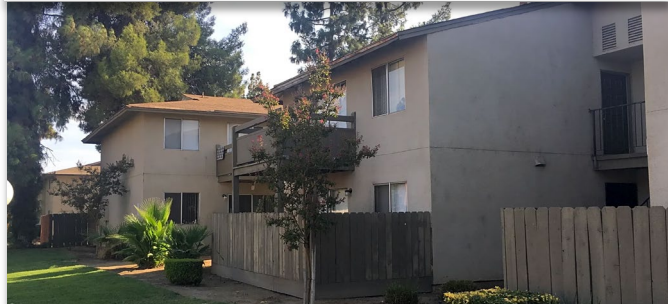
2120 Villa Ave, Clovis Ca, 93612 EDGEWOOD APARTMENTS
