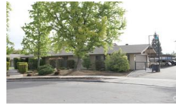
Calimyrna Apartments 502 E Calimyrna Ave, Fresno, CA
